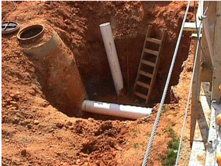
Sewer lateral going into a manhole.
