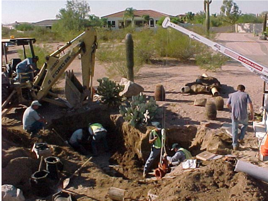
Top photograph, two gate valves blew out, you can see the kickers or thrust blocks in the back ground. Bottom photograph, a tapping machine and a new gate valve. These tapping machines are very, very expensive.
