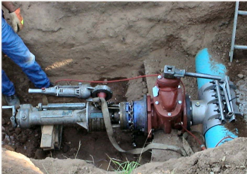
Top photograph, two gate valves blew out, you can see the kickers or thrust blocks in the back ground. Bottom photograph, a tapping machine and a new gate valve. These tapping machines are very, very expensive.
