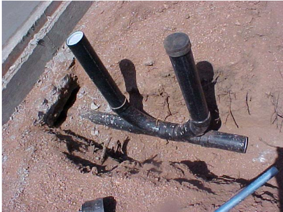
2-Way Cleanout DWV Soil Pipe, needs to be within 2 feet of the house, perpendicular (not parallel) to the footing and the end or grade level needs to be painted to protect from sunlight.
