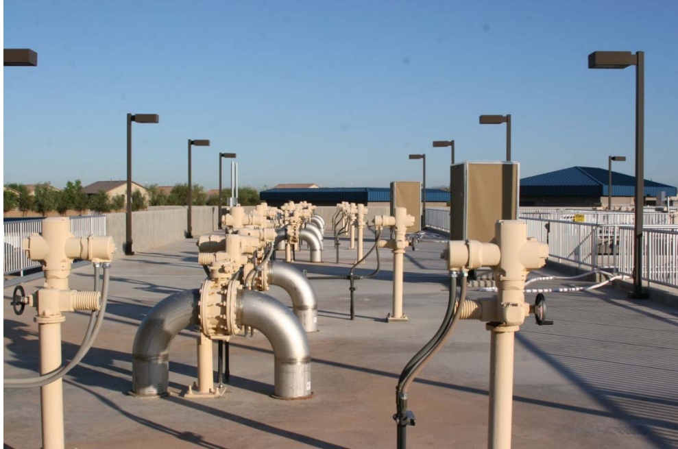
Here at a water treatment plant, we can see both valve actuators control devices and Butterfly valves as well. Bottom photograph is a cut-away of an actuator.
